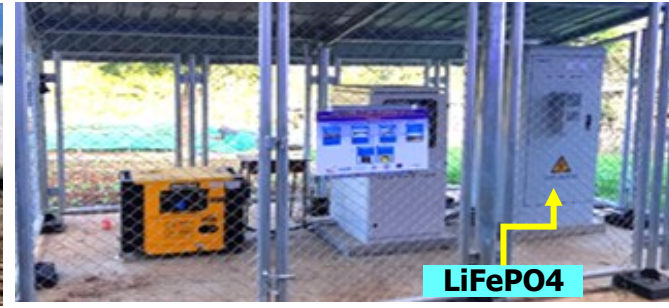
Solar Power & Battery Cabinets
