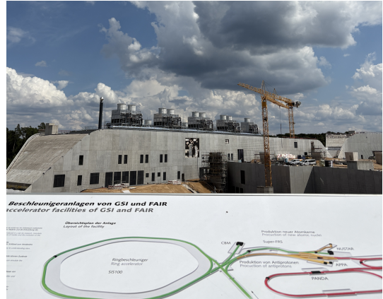
Figure 2.6: The ongoing FAIR construction site
