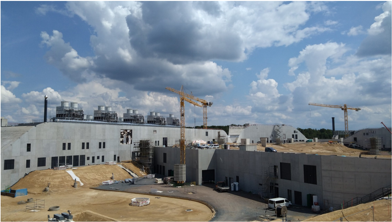
Figure 3: FAIR construction site
